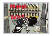
Installation no longer requires a "Trip Test", thus saving on time and equipment. The BFM-II can be powered from either AC or DC, and programming and monitoring of each circuit is possible via the display, or the built-in USB port, using SATEC's free PAS software. The information monitored is sent to the substation
