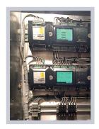
The BFM-II is designed to upgrade legacy substations featuring electro-mechanical (EM) relays, to provide realtime information and control over these highly reliable, yet limited, devices.
